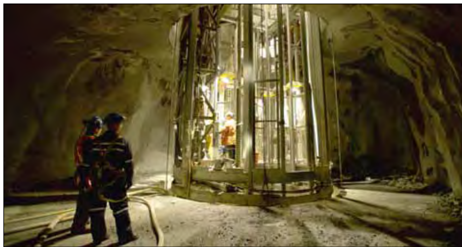
Cementation is a leader in the mine construction and engineering field.
