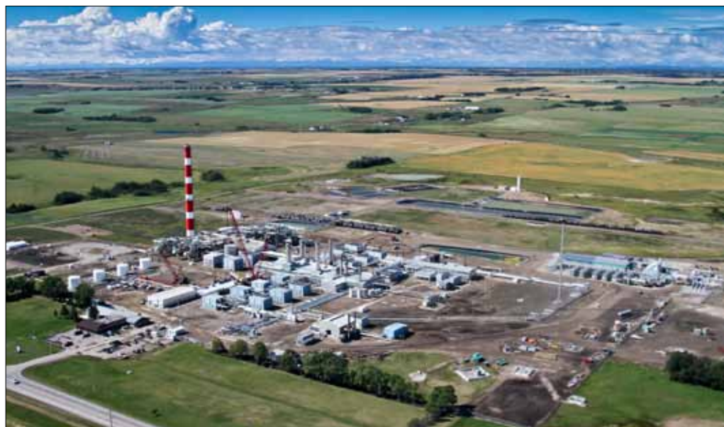
TAQA North's East Crossfield Plant.
